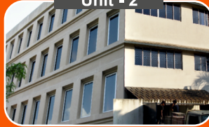
KASBA, KOLKATA Products Distribution Boards, Bus Bar, Main Switches and Change over
